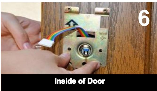
With the arrow visible and pointing up, slide the brass plate and the pigtail through the hole. **Tip: Put something in the doorway to prevent door from closing.**
