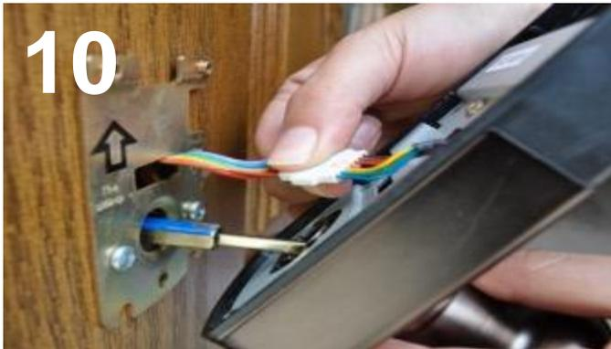
Ease the pigtail connector and excess wires into the hole as you slide the back door knob onto the blue cylinder. **Note: Lock will not work if pigtail is squashed against the door.**
