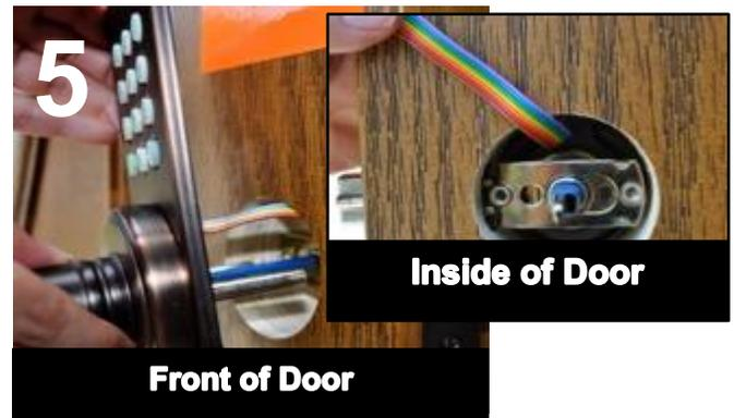
Slide knob assembly into the lower lock hole, making sure (a) the cylinder and screw tubes fit through, (b) pigtail slides in through the space above the latch, and (c) the assembly is snug to the door.
