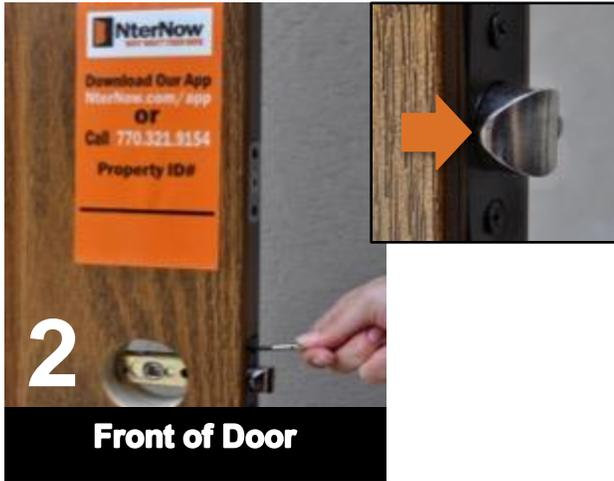
Apply front door sticker 3 ½ + inches above installation area covering deadbolt hole. Install the latch in the lower hole using the 2 flat-head screws provided. Be sure latch is in this position.
