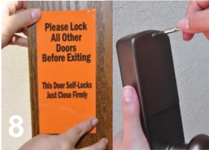
Apply inside door sticker over the deadbolt hole at least 2 inches above the brass plate. Remove the battery cover from inside knob assembly and set the small screw aside.
