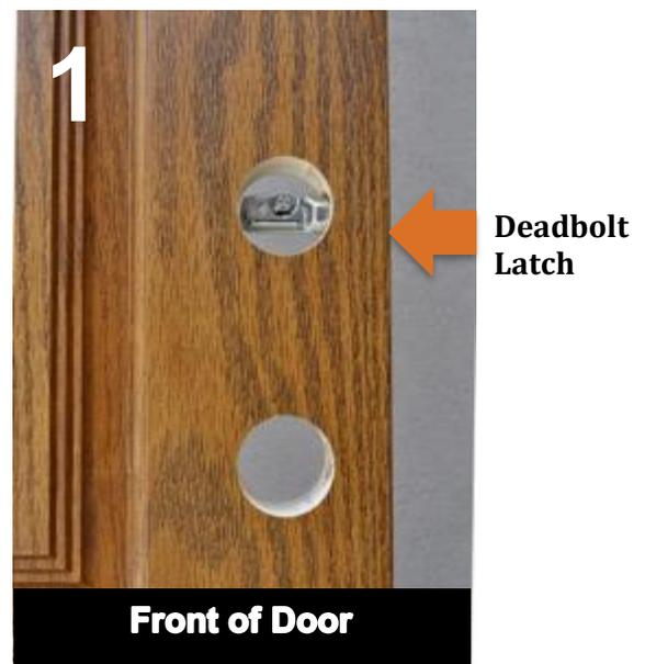
Remove all the current lock hardware on the door except for the deadbolt latch.
