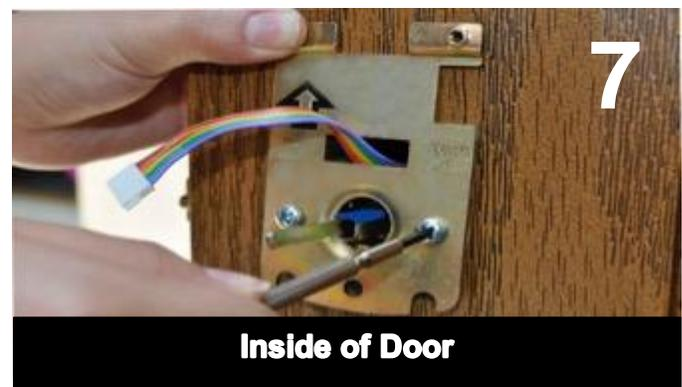
With one hand squeezing the front door knob assembly and the plate together, rotate the 2 silver screws into the screw tubes. Once screw grabs, tighten it with the accompanying screwdriver. **Tip: Do not use a power screwdriver -- it will over-tighten!**
